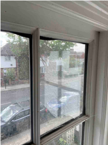
Timber windows to front elevation - failed DG units and condensation damage to timber framing
