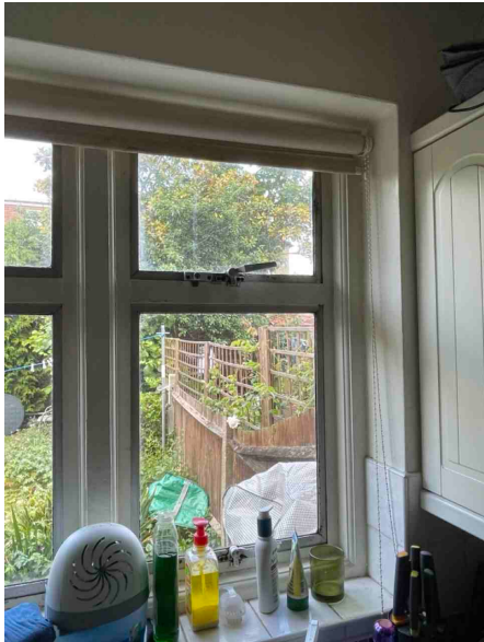
Aluminium framed glazed units set within original timber framing - condensation damage and mould growth
