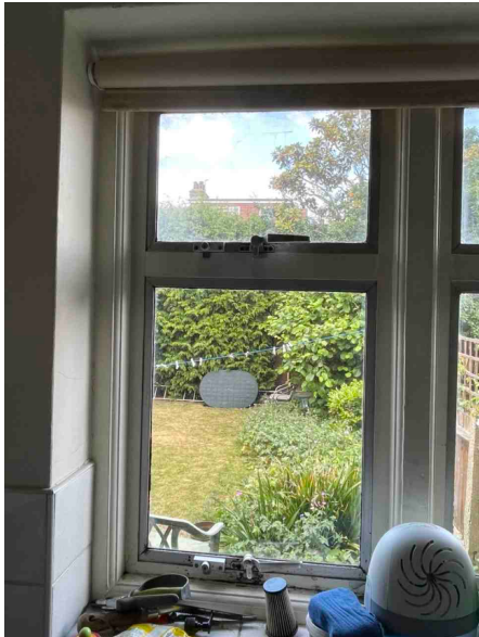
Aluminium framed glazed units set within original timber framing - condensation damage and mould growth
