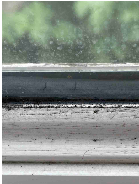
Timber windows to front elevation - failed DG units and condensation damage to timber framing
