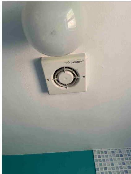
Loft hatch - not sealed or insulated. Basic iMEV in bathroom and kitchen
