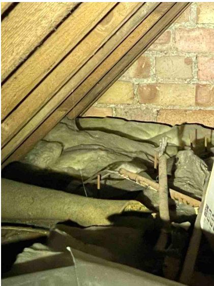
Inconsistent roof insulation between joists, uninsulated rafters
